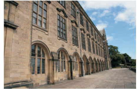
The Main Arts Building Terrace
